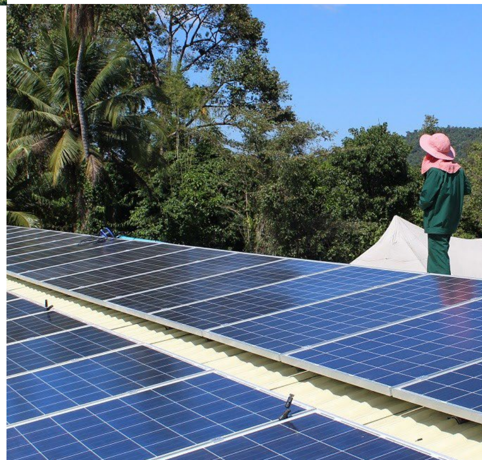
A worker inspects the solar panels installed by Solar Green Energy in Cambodia.
