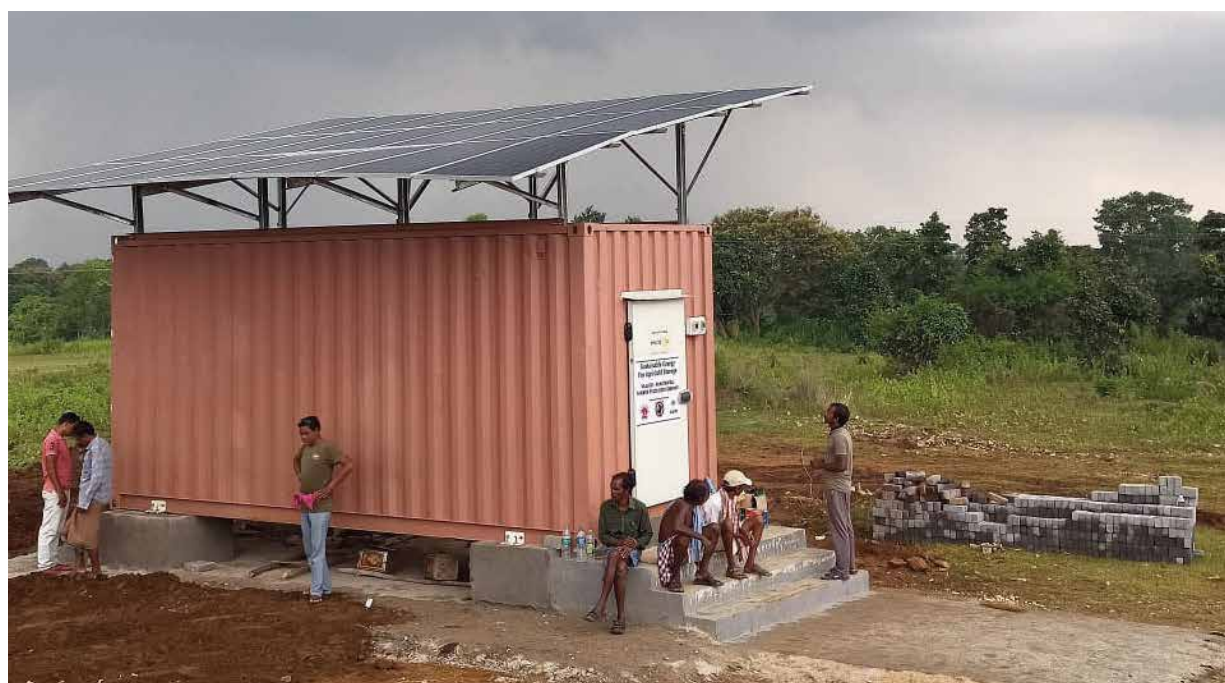
Right: Inficold solar cold storage for agricultural produce by Sanatanpali Farmer Producer Company in India.
